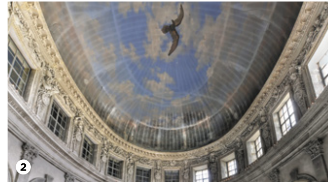
2. Restoration of the Great Cupola in the heart of the Château.
